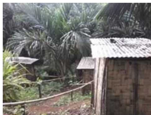
VIP toilet at Haren Hala School
