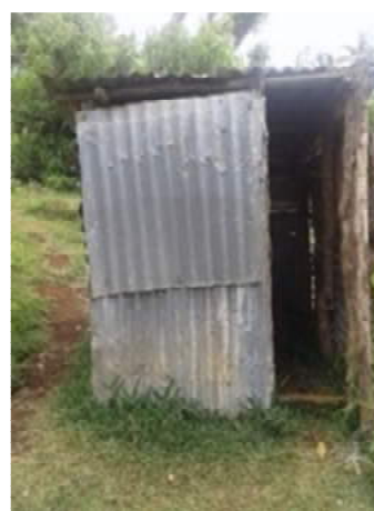
Toilets at Lalzadeth Primary School, the school are now in the process of getting some new improved toilets for its students.
